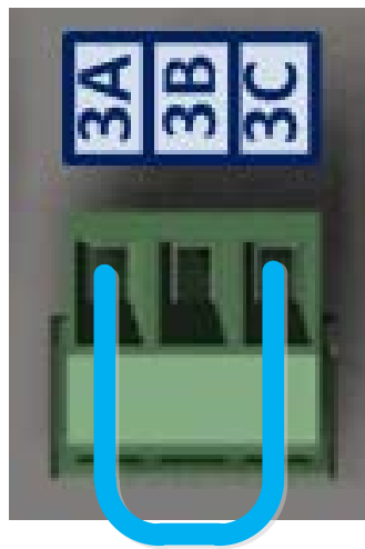
Fig. 20 VVVF Drive supply output and Inverter V230ac output external enabling (Short-circuited - ON / Open-circuited - OFF)
